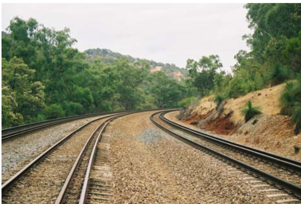
Figure 6 : A location where off-train communication is difficult. The terrain will limit coverage to the rear of a train on this curve.
