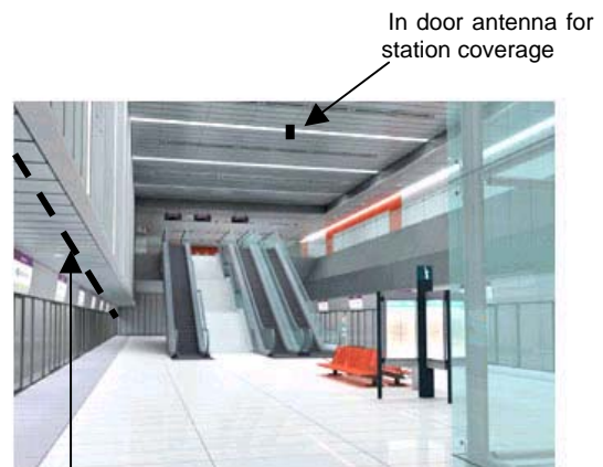
Figure 9 – Position of antenna and LCX cables on the ceiling of a typical MRT station
