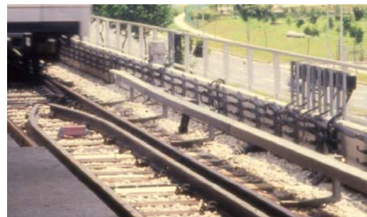
Figure 2: IRJ Block Termination on Sleepers
